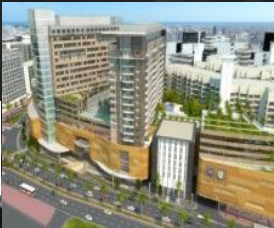
Al Khor Rayhaan Hotel 428 Rooms
